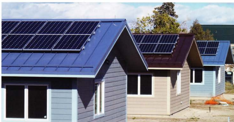
PV and solar thermal installation by Creative Energies of Lander. Photo courtesy Scott Kane.
