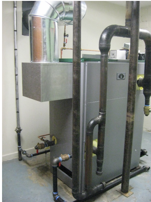
Figure 24. Niobrara County Library, Lusk, new furnace
