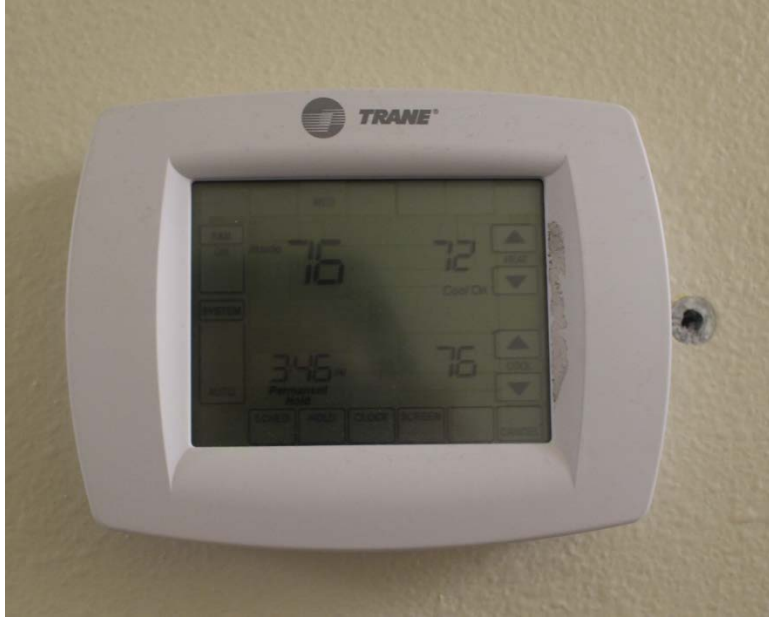
Figure 19. Goshen County Public Health, Torrington, programmable thermostat
