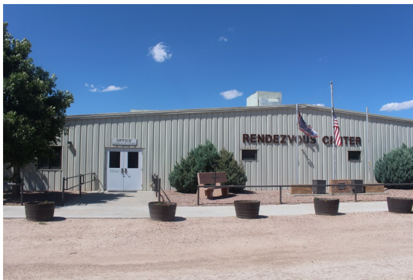
Figure 12. Goshen County Fairgrounds Rendezvous Center exterior, Torrington
