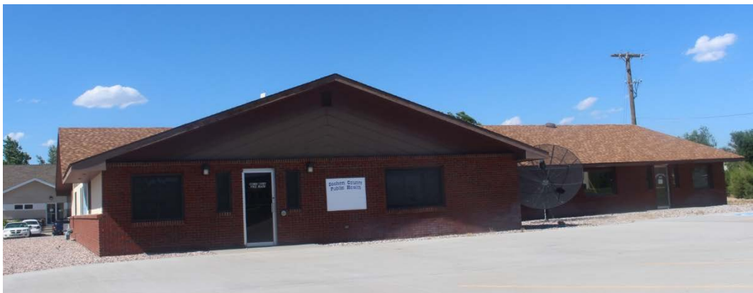
Figure 17. Goshen Public Health exterior, Torrington
