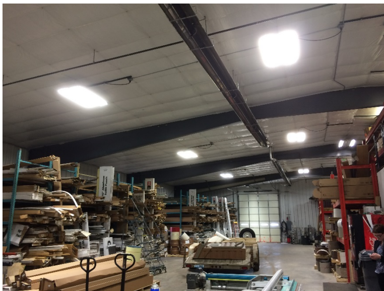
Figure 2. ABC Seamless warehouse, Cheyenne, after lighting retrofit
