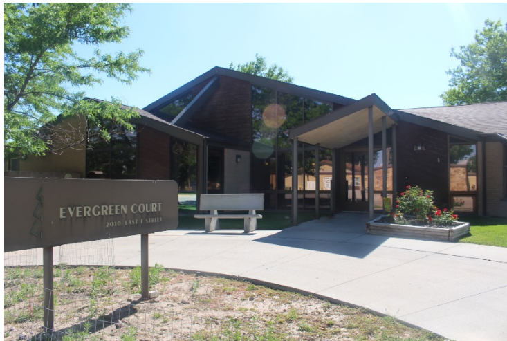
Figure 7. Goshen County Evergreen Court exterior, Torrington
